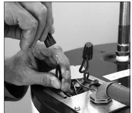
Figure 19 - Connecting the electrical wires.
