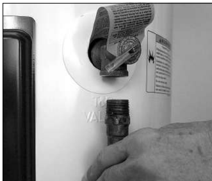
Figure 11 - Removing the T&P Relief Valve discharge pipe.
