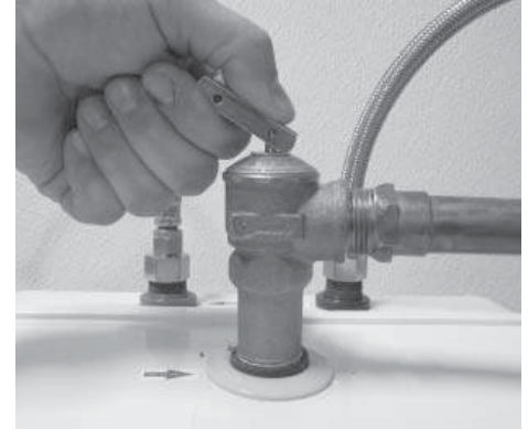
Figure 31 - T&P Relief Valve
