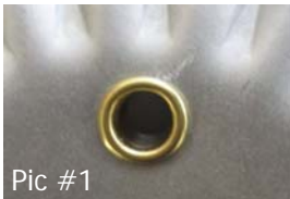
Drip hole in burner
